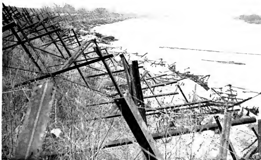
Fig. 3—After silting has become established.
